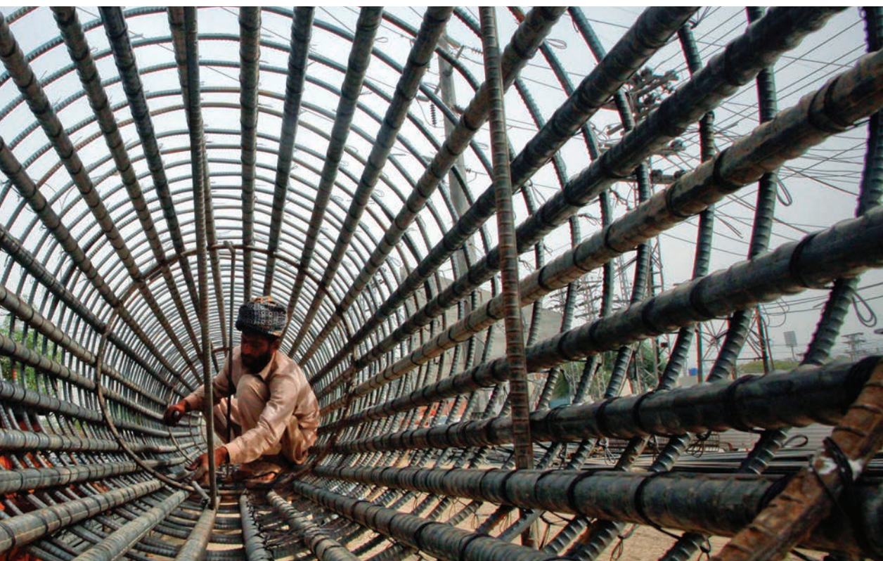
< A labourer attaches iron rods to a column at the construction site of a flyover in Lahore. REUTERS/ Mohsin Raza
